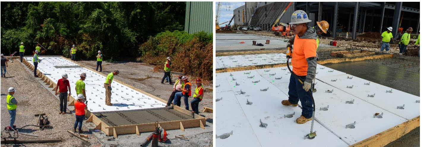
Photo on the left: walking in foam. Photo on the right: walking in foam and vibrating IconX connectors.
